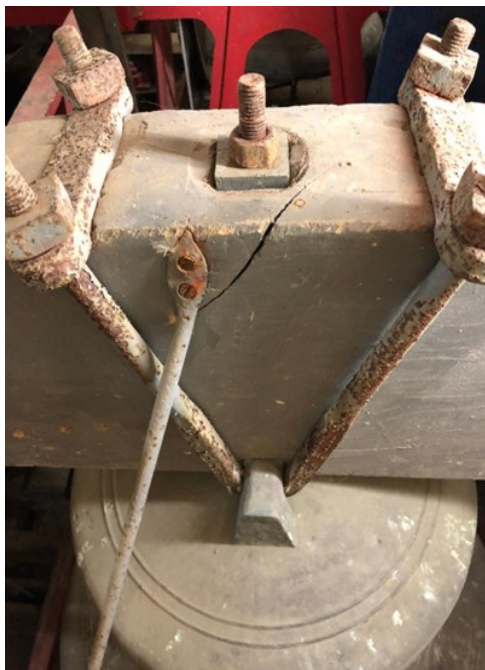
The cracked wooden headstock on the 6th
