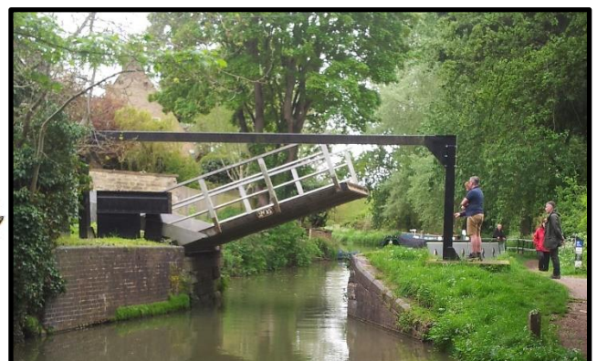
One of many lift bridges.
